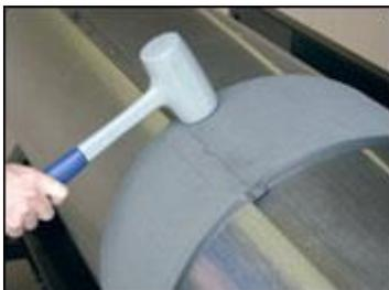
The final hammer blow should be delivered near the edge of the cover, just above the seam.
